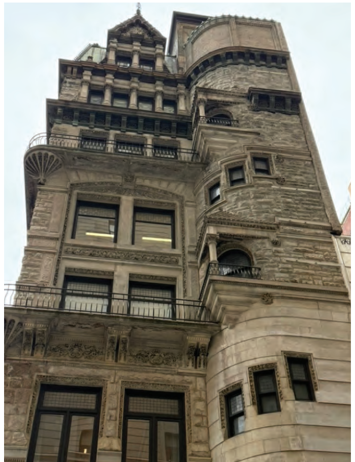
Detail of the Chestnut Street façade of the Hale Building as it looks today
