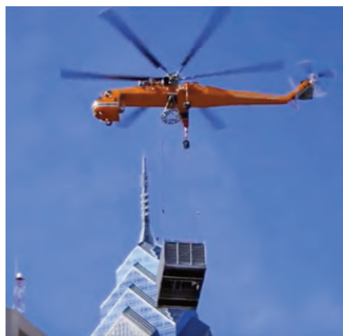
Sikorsky Skycrane lifting an HVAC unit
