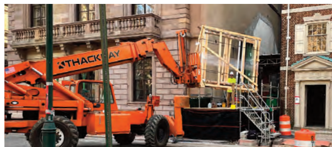
A telehandler lifting window glass at the Dilworth House
