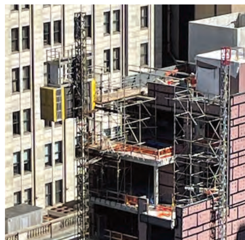
A buck hoist at work at the Dilworth House
