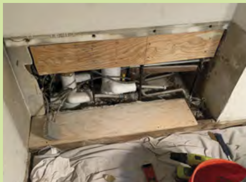
Fan coil removed.
