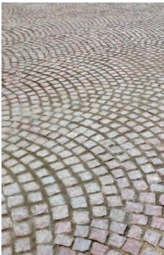
The brick pavers had to have grout patted down manually
